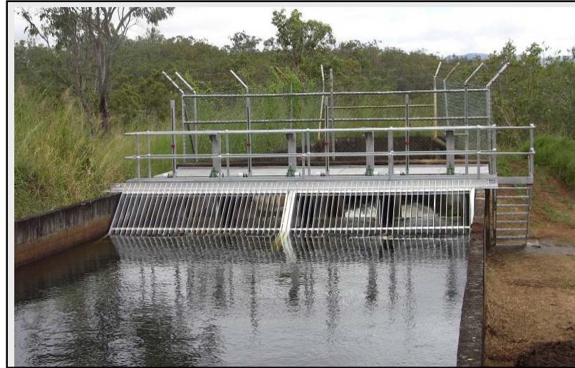
Trash Rack at Outflow
